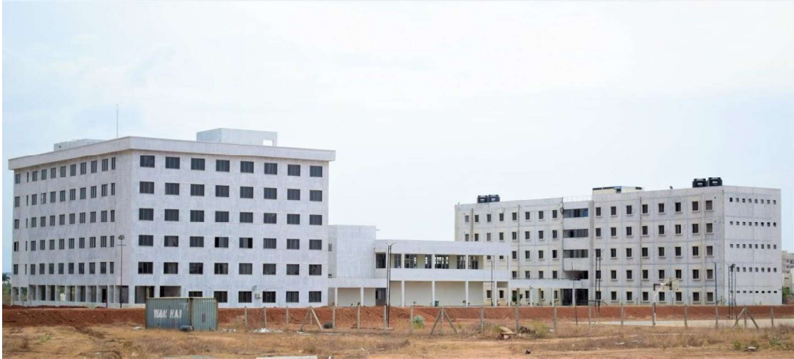
Hostels and Dining Hall Facility
